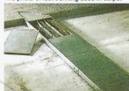
易安线槽与地毯面使用图例 The photo of fast trunking used in carpet
