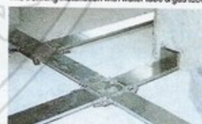
线槽交叉及引上安装 Trunking across & line up installation
